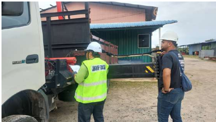
LORRY CRANE INSPECTION BY DOSH 3.4.2025
